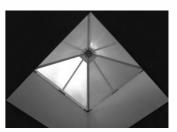
Using angular selective skylights. It can filter sunlight with high incident angle
