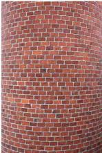
Above (left): Steel used in roofing Above (right): Granite plinth Left: Chimney's header bond Below: Load bearing walls in English Bond
