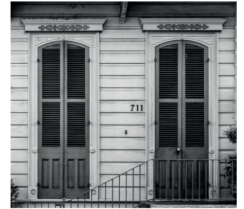
Figure 34: shutter over door and window in a shotgun
