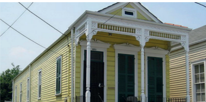
Figure 40: a single shotgun with symmetrical facade, porch and gable roof
