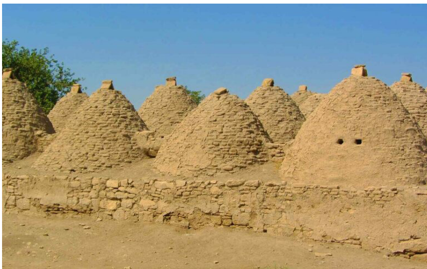
Figure 5.10: [left] Adobe brick material in construction (Cortesi, 2020)
